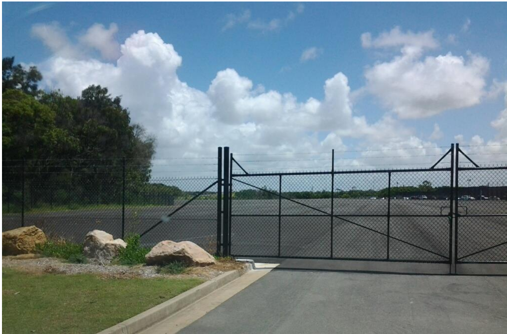
Figure 3: Former public access road to the former Visitors Centre.
