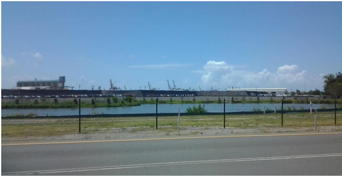
Figure 4: View of the former Visitors Centre site, showing paving right to the water's edge.
